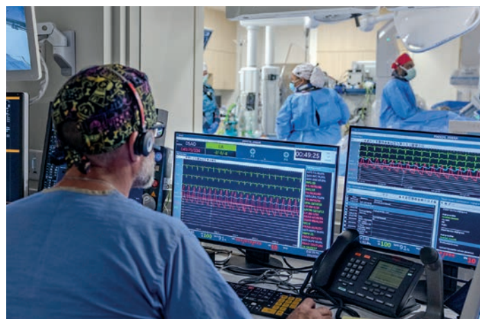
The new cath lab also has additional cameras and communications systems, as well as extra cameras to perform live cases and train other physicians.
